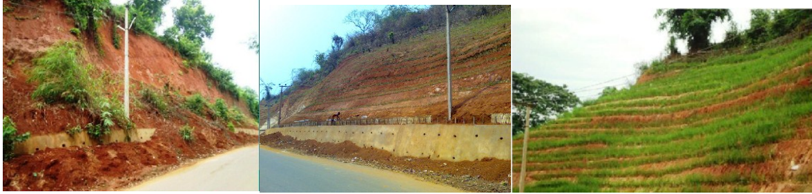
Figure 6 Slope before plantation, plantation of vetiver and after 3 months.
