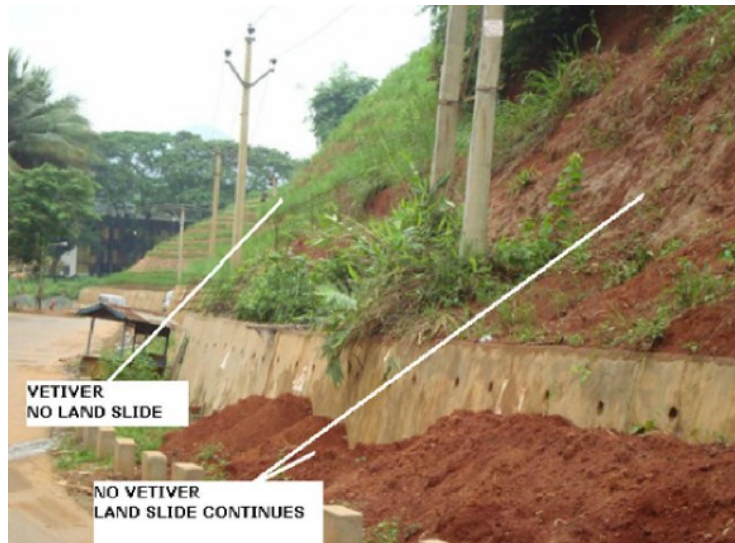
Figure 7 Effect of vetiver in preventing erosion and slope failure.
